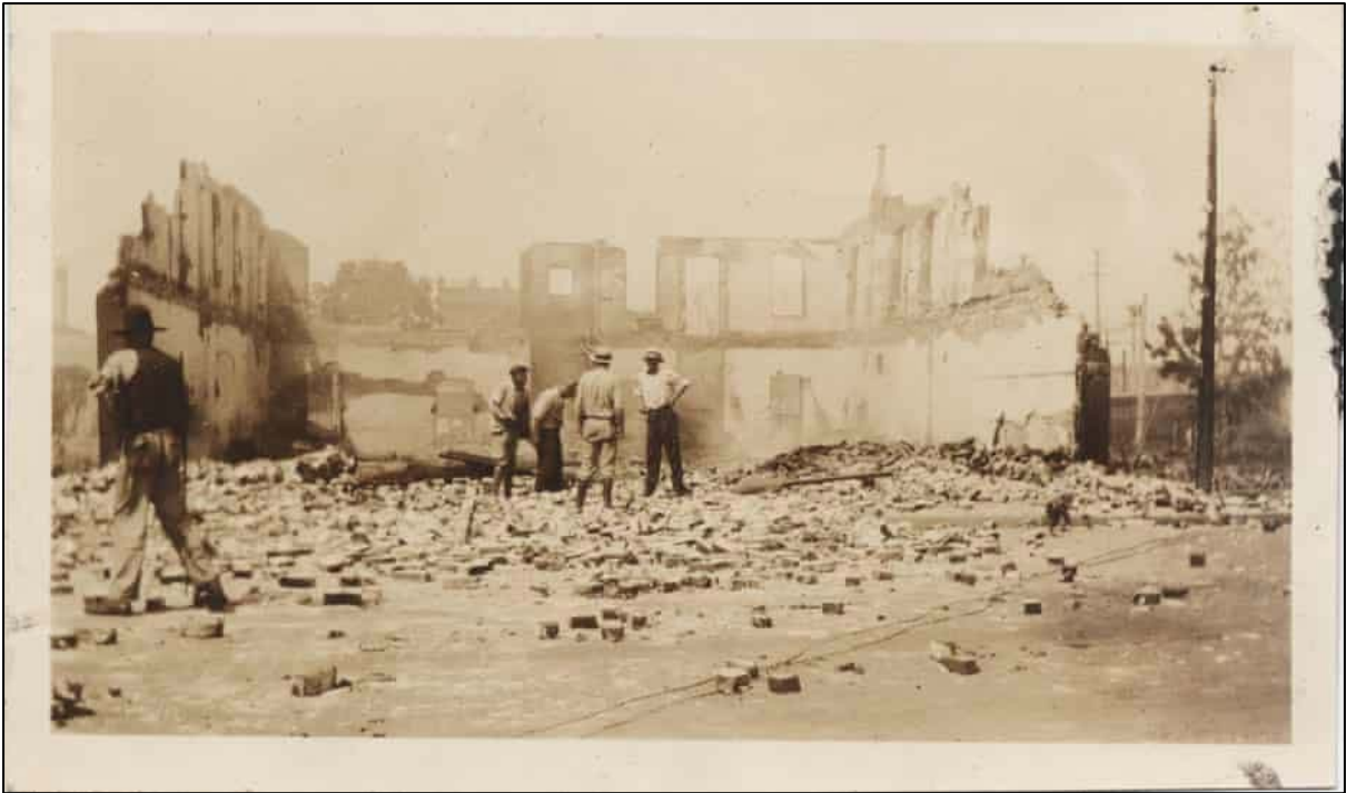
Black Tulsa residents stand in front of a leveled building in Greenwood.
